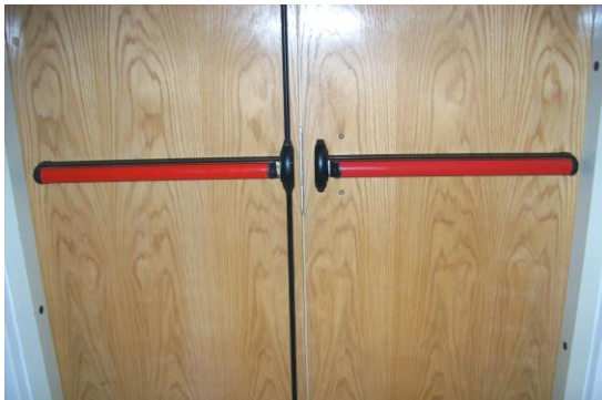
DOUBLE DOOR SOLUTION with panic hardware on each door, key bypass and electronic access control
