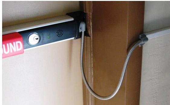
Door loop is used as shown above to conceal the cable
